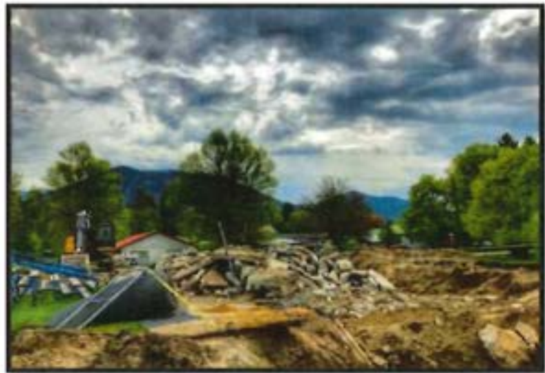
Swimming Pool Demolition
